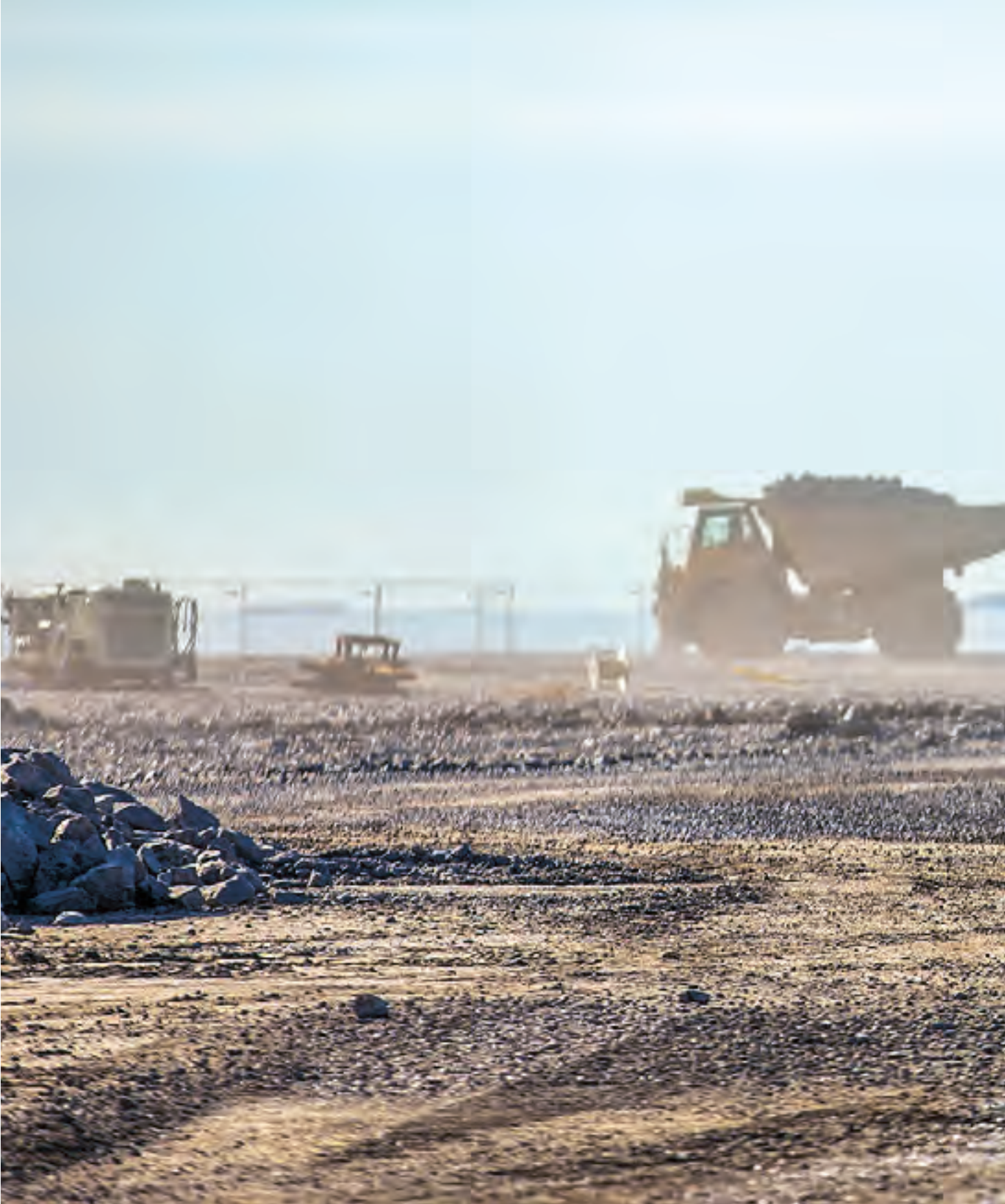
Watering | A water truck constantly sprayed the ground in the emerging port area to keep hazardous dust to a minimum.
