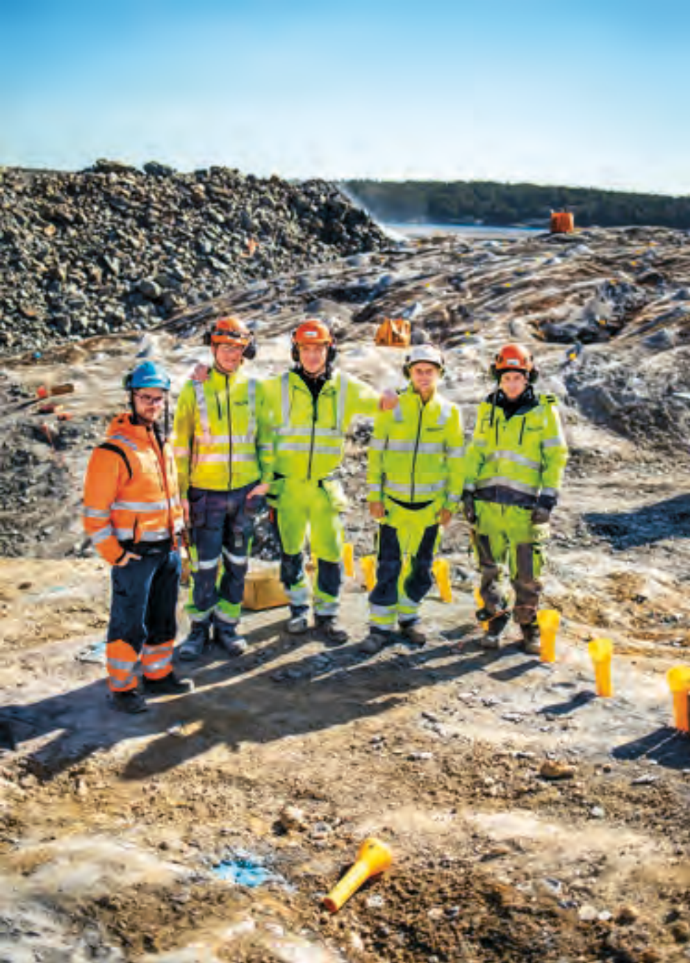
The big blast (left) | The biggest blast removed 351,000 tonnes of rock to make room for the railway yard. It took 475 bore holes and almost 100 tonnes of explosives to remove so much rock. This was the largest rock extraction ever in Sweden, outside of mining.
